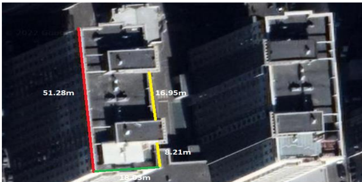
Figure 16. Olympic residence rooftop
