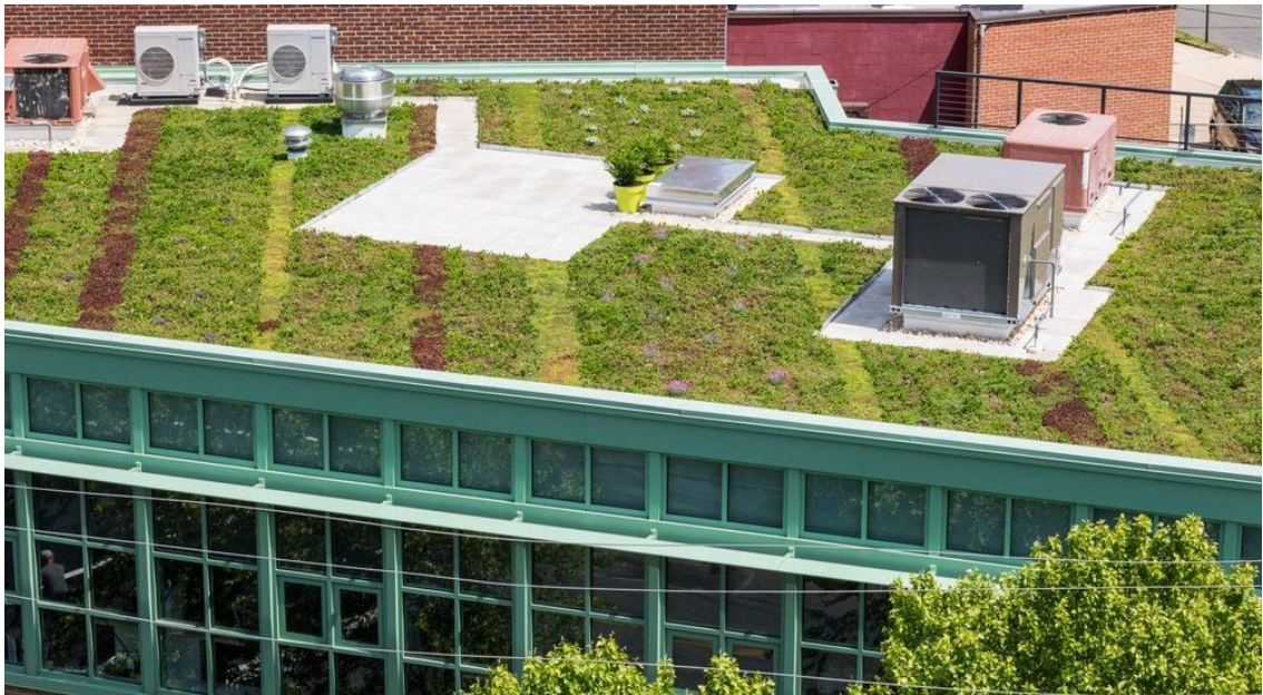
Figure 1. General green roof on a residential building
