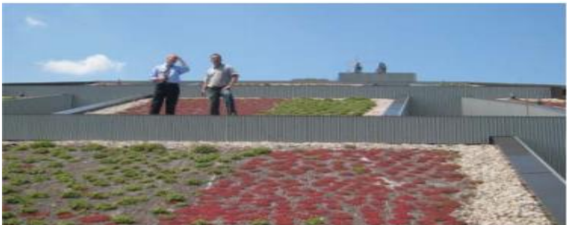
Figure 5. Flat green roof
