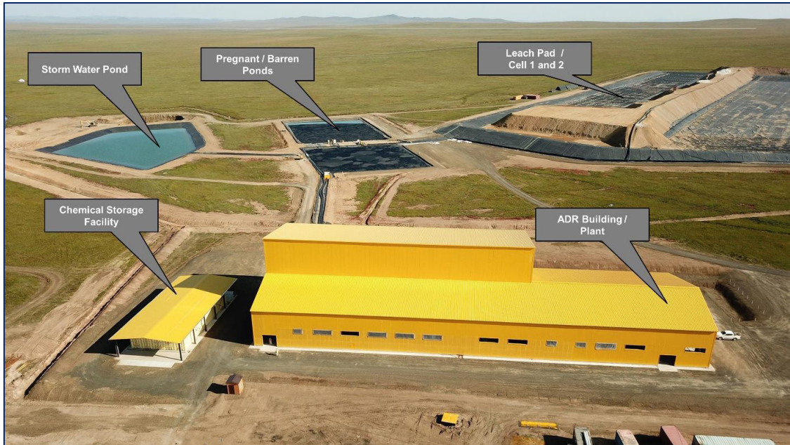
Figure 15. Process plant layout of ATO project
