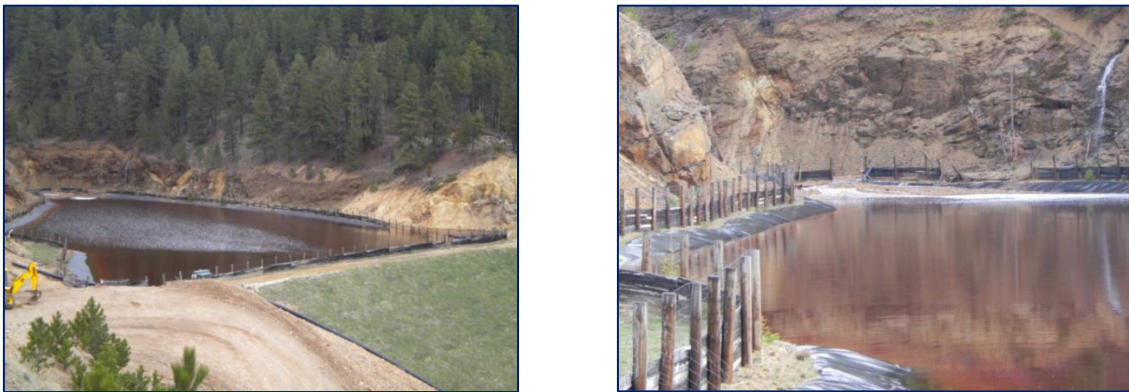
Figure 24. Overflowing the capture pond of Zortman mine (68)
