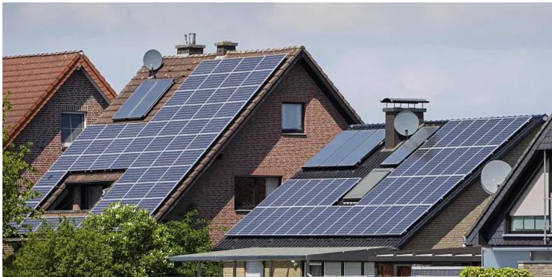
Figure 1. Rooftops PV systems on private houses, Duelfmen, Germany
