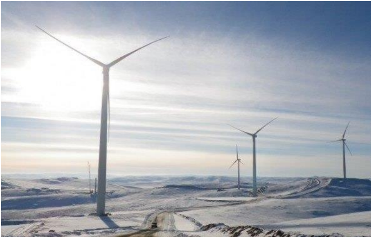
Figure 9: Salkhit wind farm (11)
