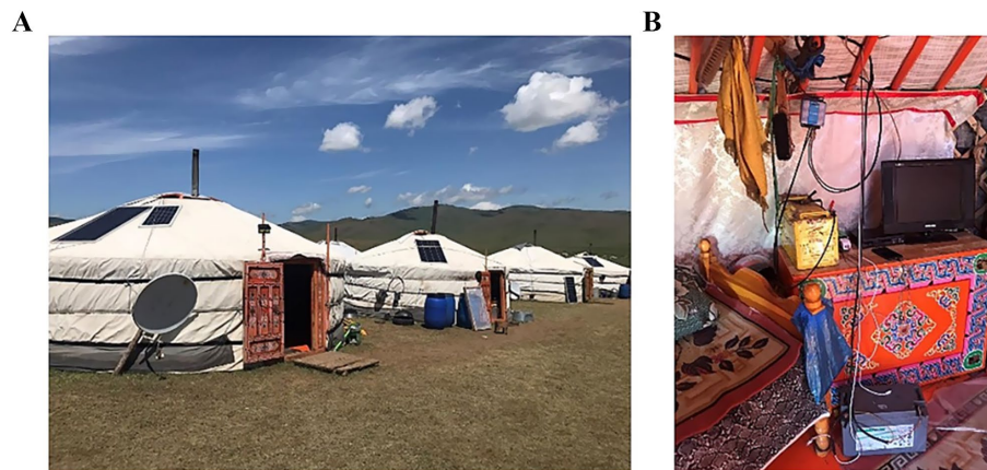
FIGURE 10 Solar panels used in Mongolian gers (A) and lead acid batteries used as energy storage systems (B). Source: Prates et al. (2023). (authors' own archive).
