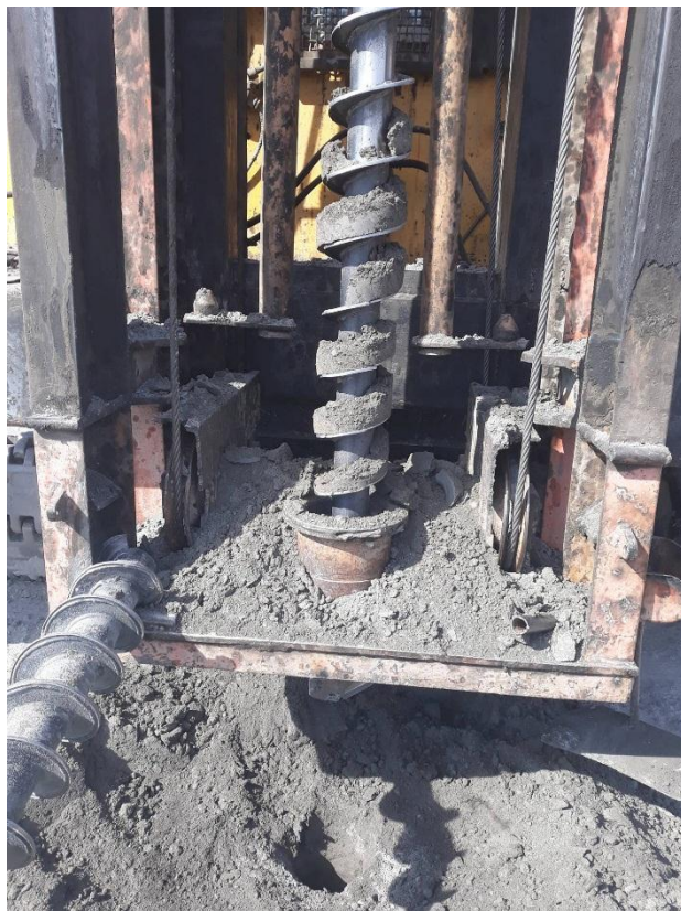
Figure 1. 5 – Borehole drilling (SBR-160A-24)
