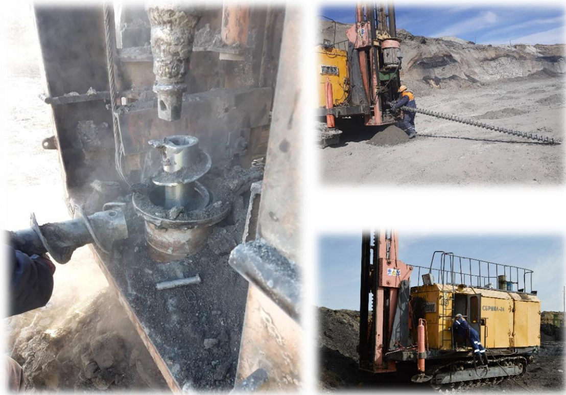
Figure A. 2 - The drilling rod extending process
