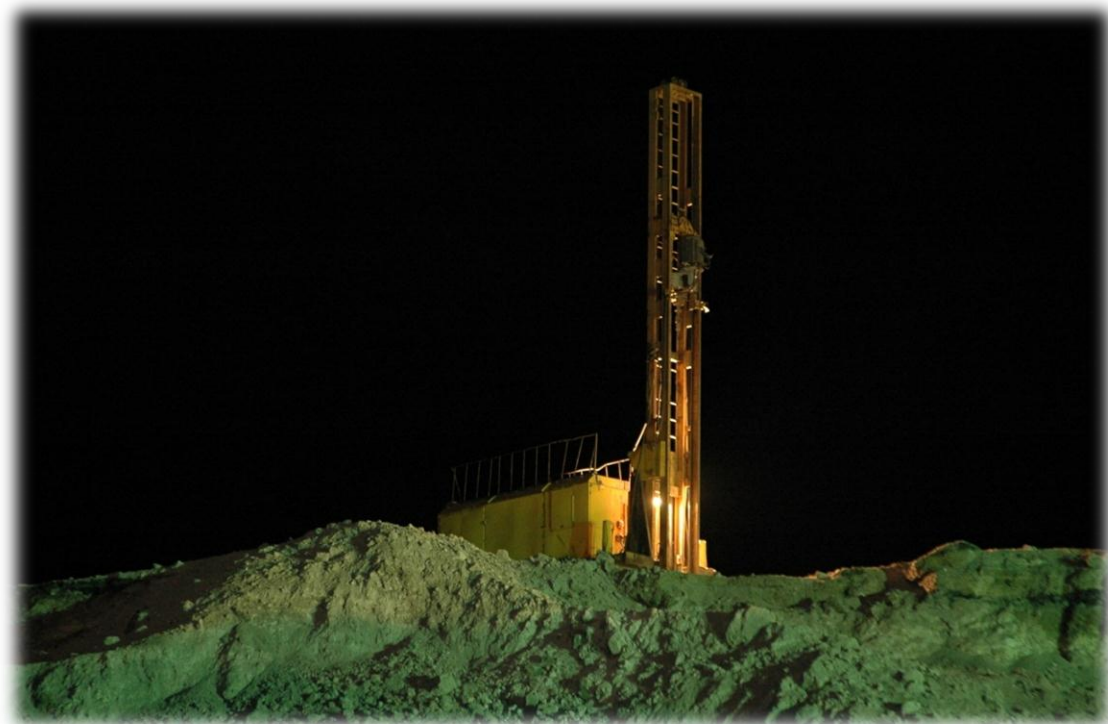
Figure A. 3 - The auger drilling rig (SBR-160A-24)
