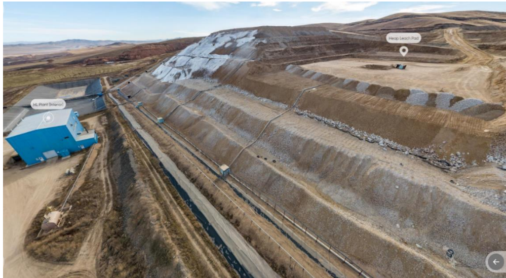
Figure 20: Heap construction of Boroo Gold LLC.
