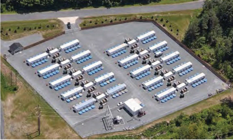
Figure 4.27 A flywheel-based storage plant for frequency control (20 MW/5 MWh). Source: Beacon Power, LLC, 2015 [169]. Reproduced with permission of Beacon Power, LLC.
