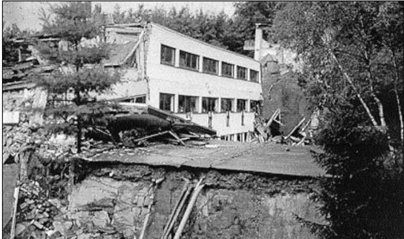
Figure 8 Children's hospital damaged by underground mine subsidence in Oppenheim, Germany (13)
