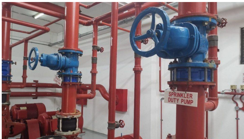
Figure 21. Sprinkler Pump
