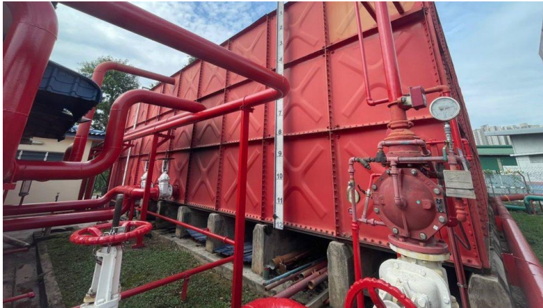
Figure 23. Sprinkler Tanks
