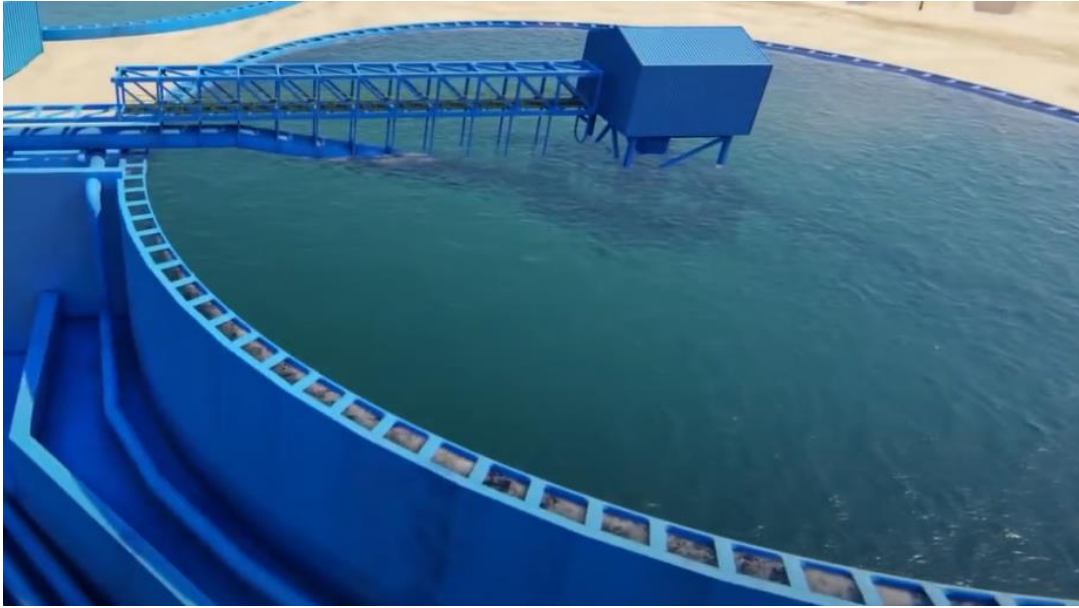
Figure 8: Thickening the tailings at Oyu Tolgoi concentrator [4]
