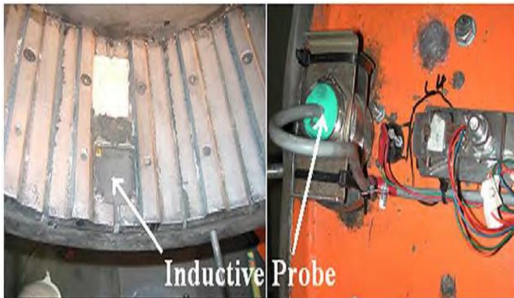
Figure 2. 15 – Installation of the Inductive Proximity Probe on the Pilot mill
