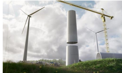
Figure 2: Tubular steel wind turbine tower
