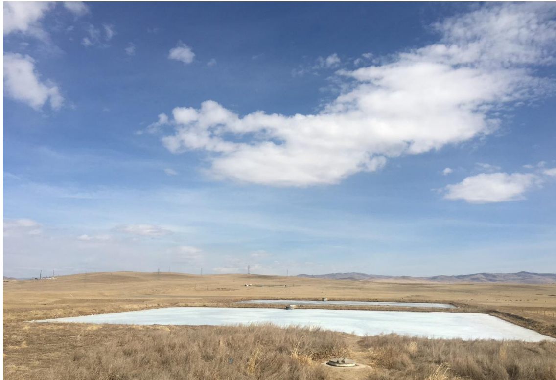
Figure 4: Polising pond of Gorodok WWTP
